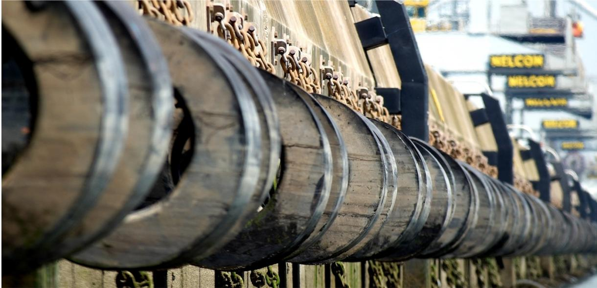
**Figure 2: Cylindrical fenders at Delta Terminal Rotterdam (photo PoR)**
