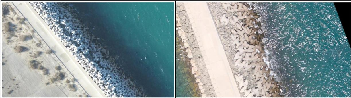
**Figure 6 Impression of (local) damages after TC Gonu**
