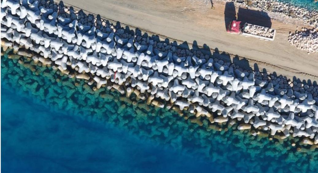
**Figure 14. Prototype Tetrapod placement pattern**
