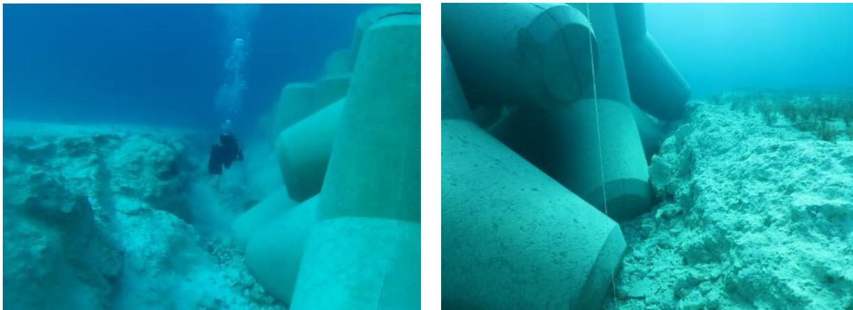
**Figure 13. Prototype excavated trench and confinement of Tetrapods by the trench at the shallow section.**
