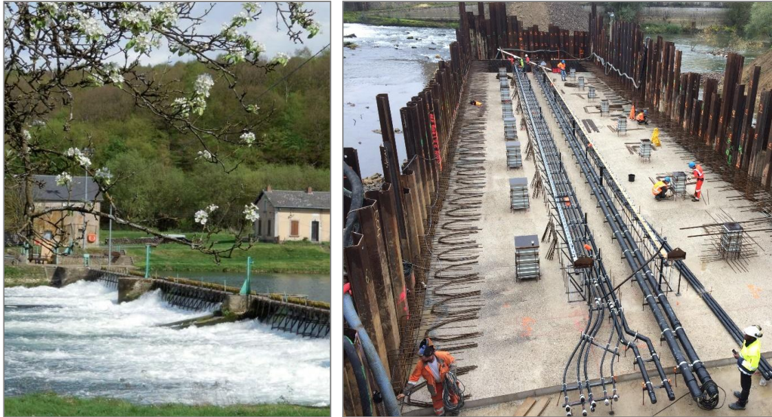
Figure 3: Montigny existing weir on Meuse river (left) and construction of Mézières dam on Meuse river, without reusing piers and abutments (right)
