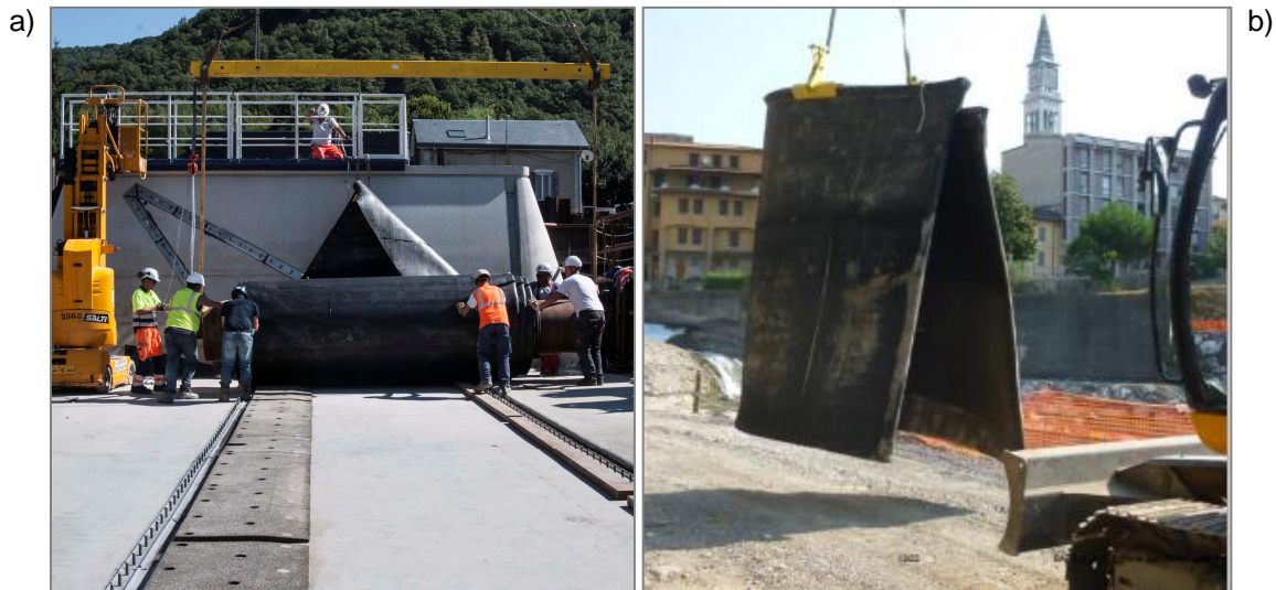
Figure 4: Handling of a) membrane for Rubber Gate and b) bladder for SR Gate
