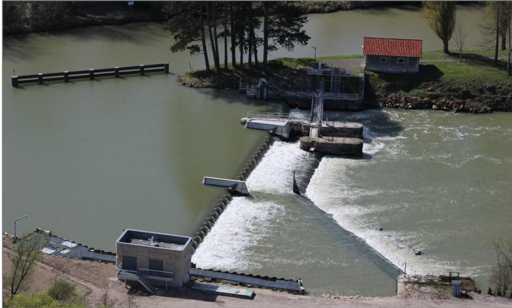
Figure 5: Carandeau two-span weir (Aisne) the old weir and its piers have to be demolished
