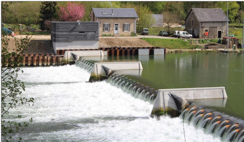
Figure 6: Montigny three-span weir (Meuse) and its new control house
