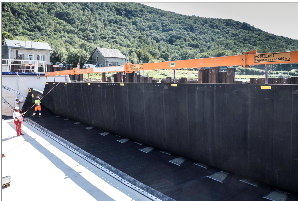
Figure 1: Installation of a rubber membrane
