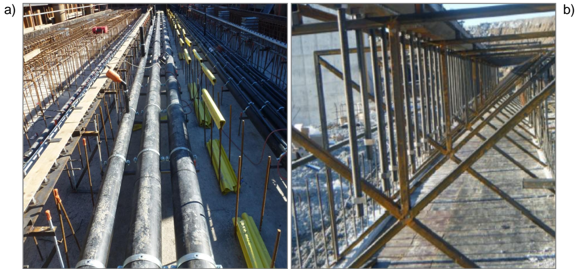
Figure 3: Installation of embedded parts for a) Rubber Gate and b) SR Gate
