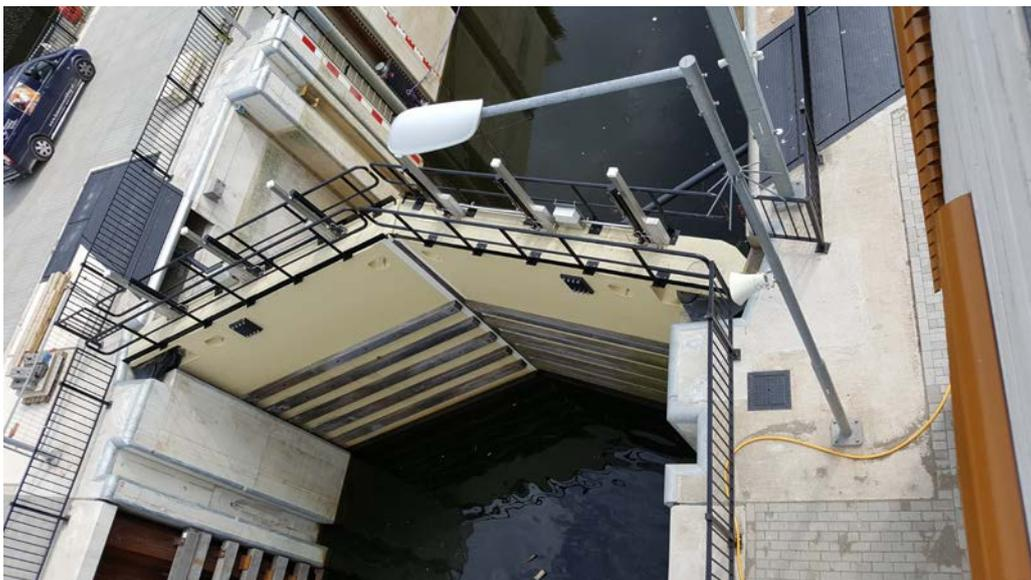
Figure 8: World’s Largest FRP Composite Miter Gates at Lock III in Tilburg the Netherlands.
