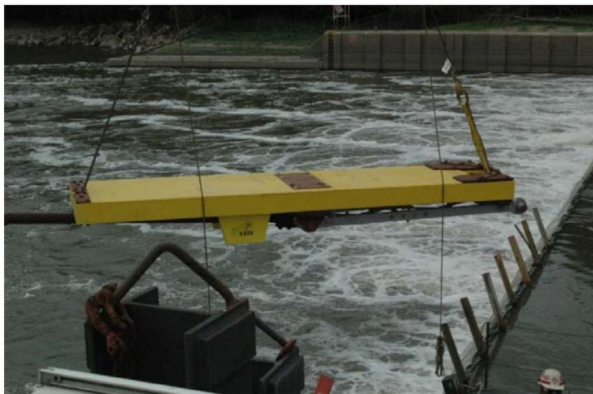
**Figure 7: Installation of FRP Wicket Gate with UHMWPE**
