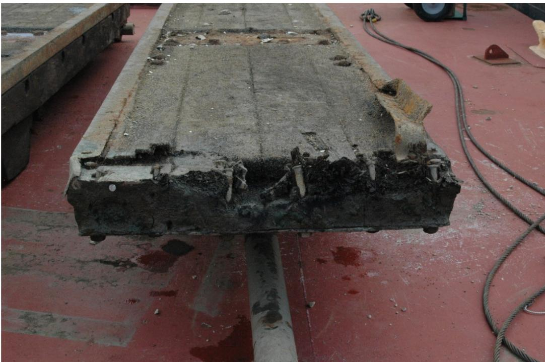
**Figure 4: Deteriorated Timber Wicket Gate**
