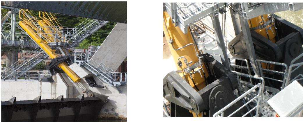
Figure 13 Hydraulic cylinders - vents downstream of the gate - cardans joints
