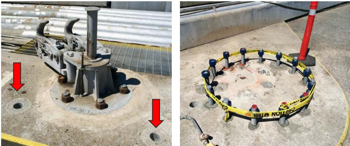
**Figure 2: New mooring hook installations showing preinstalled coring for anchor bolts (left, arrows) and new bolt pattern prior to setting the new hook assembly (right).**
