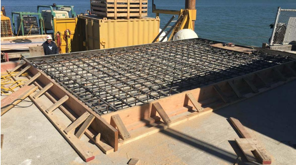
**Figure 3: An example of localized deck strengthening in preparation to support a new quick-release mooring hook on an existing wharf deck.**
