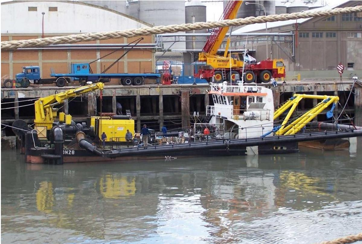
Figure 4: Dredging of the piers, wharfs and quays was done by a water injection dredge (WID).
