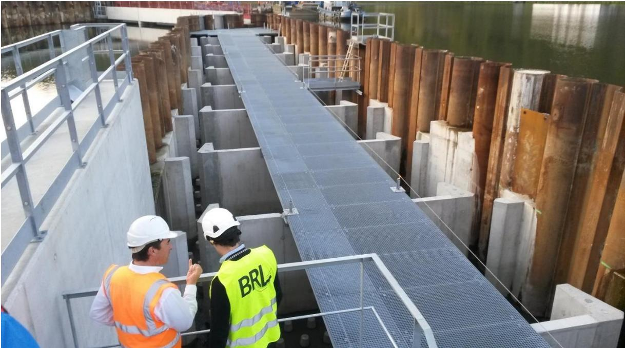
Lock 51 Saint Joseph. Fish pass of the double vertical slot type with bed substrate
