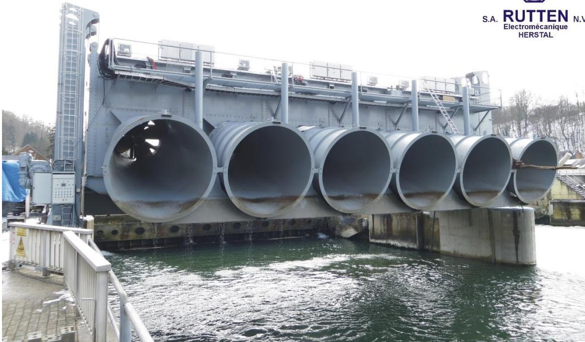
Lock 1 Hastiere showing six turbines raised up above the water to allow unrestricted flood passage.
