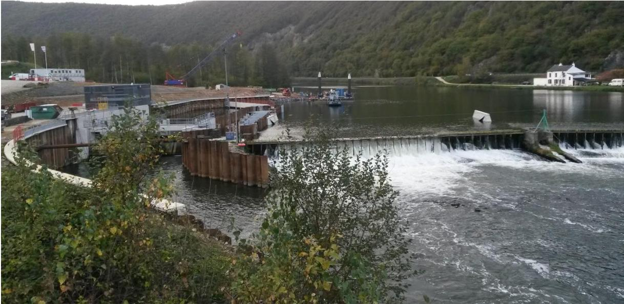
Lock 51 Saint Joseph. New channel for hydro power and fish pass on the left with the existing stake weir still in place during the construction phase.
