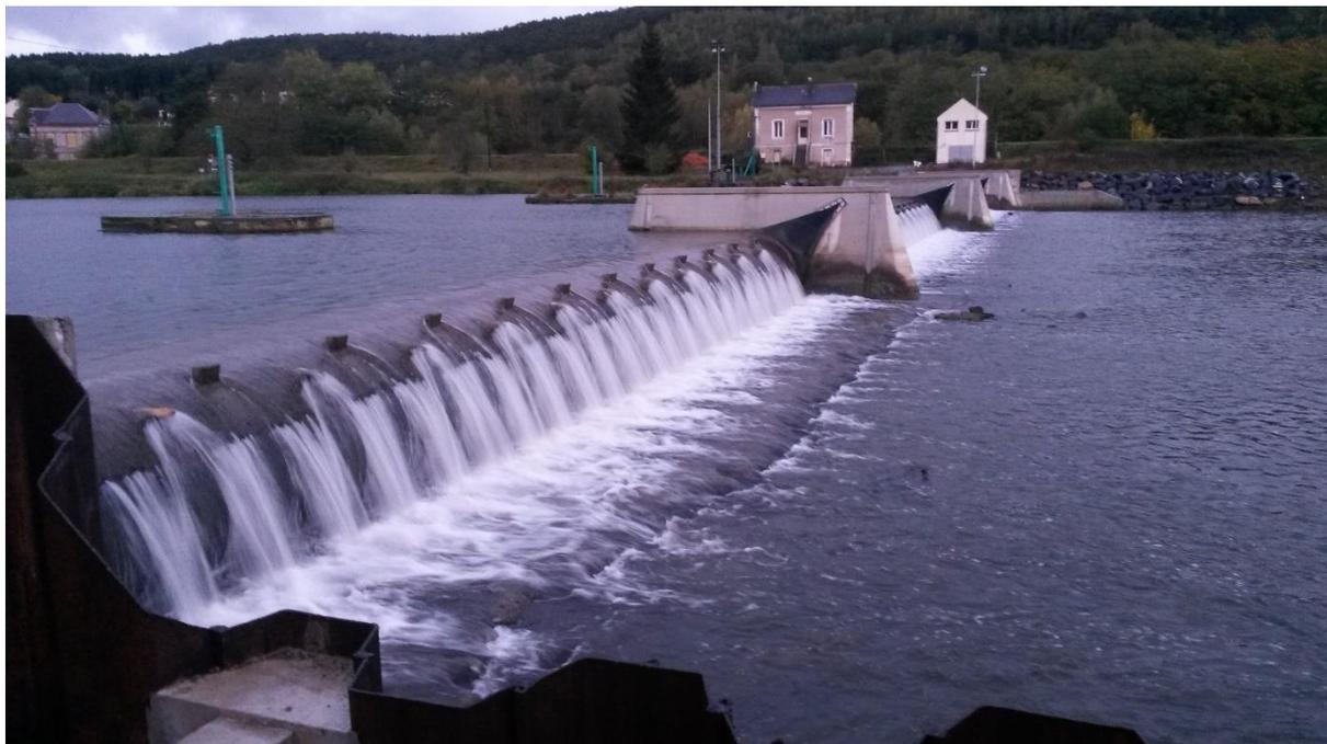
Lock 57 Ham. Inflatible rubber weir in operation. The original stake weir has been removed. It was further upstream of the new weir and its position is marked by the piers still visible.
