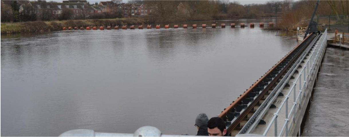
Knottingley Hydro Plant, Aire & Calder Navigation. Showing the large intakes necessary and the screen wiper at the upstream end.
