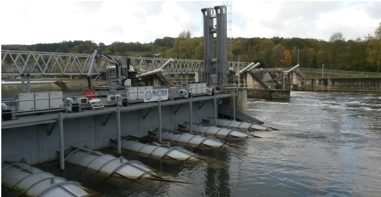
Lock 1 Hastiere showing six turbines mounted on a steel deck immediately in downstream of the weir gates. The vertical tower is part of the lifting equipment that lifts the deck clear of the river in times of flood.
