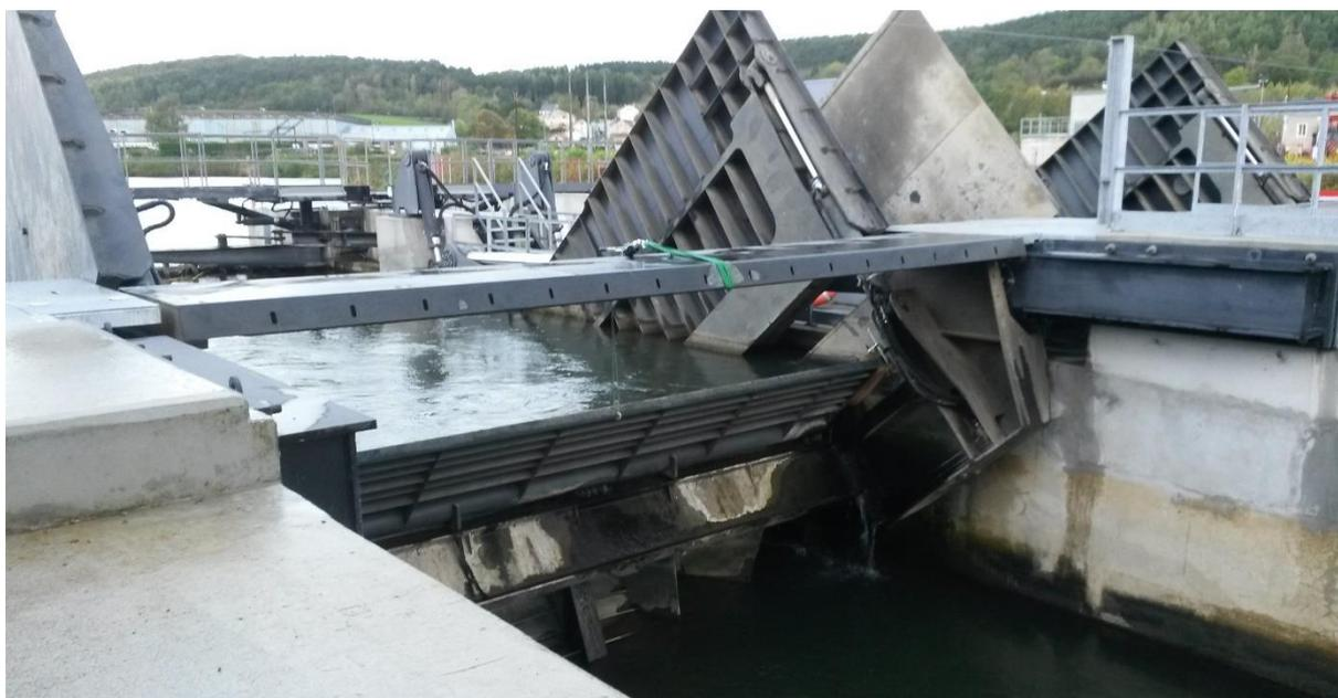
Lock 57, Ham. Very Low Head turbines in operation. In times of flood, the turbines are lowered down and the doors are closed over the turbines to allow the full area to be used for flood discharge
