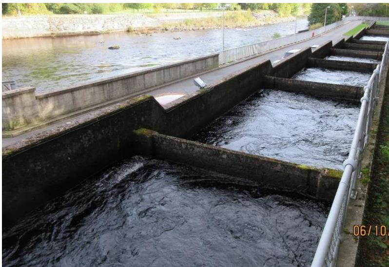
Pool fish pass in Scotland with submerged orifice
