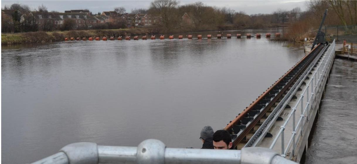
Large intake screens parallel to the main river flow on the Aire & Calder Navigation in England. These screens have the 6 mm bar spacing shown above and a horizontal automatic rake that pushes the debris into a debris chute. The picture illustrates the large size of the screens in relation to the hydro power plants output of 500 KW.
