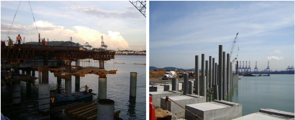
Figure 4: Phase 1 Quay Deck Construction
