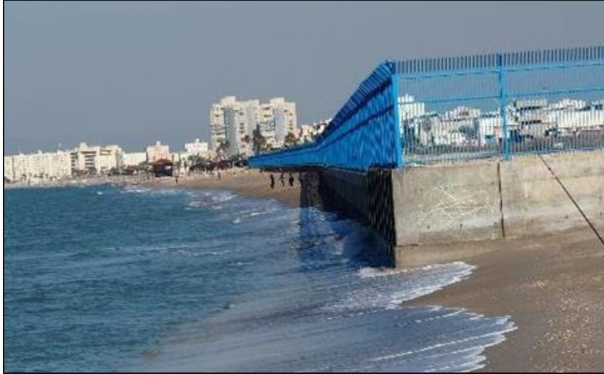
**Figure 27: Beach width in front of concrete fence before sand nourishment**
