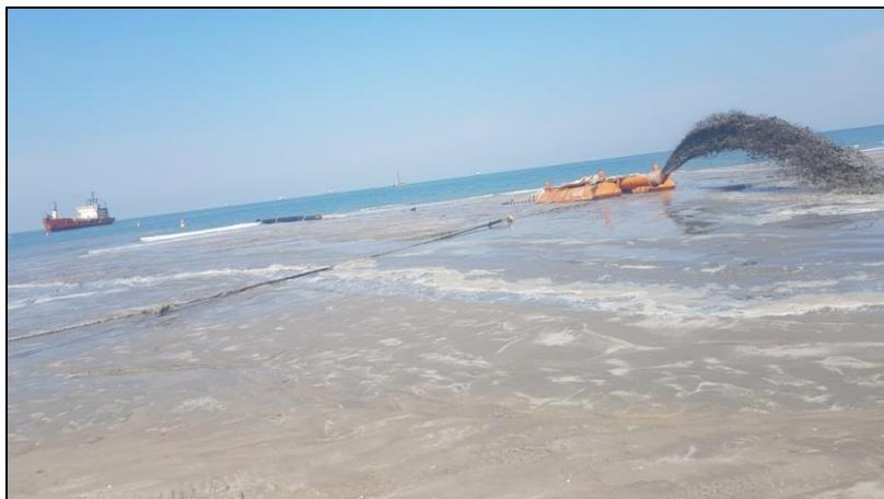
**Figure 26: Trailer suction hopper dredger pumping sand ashore**
