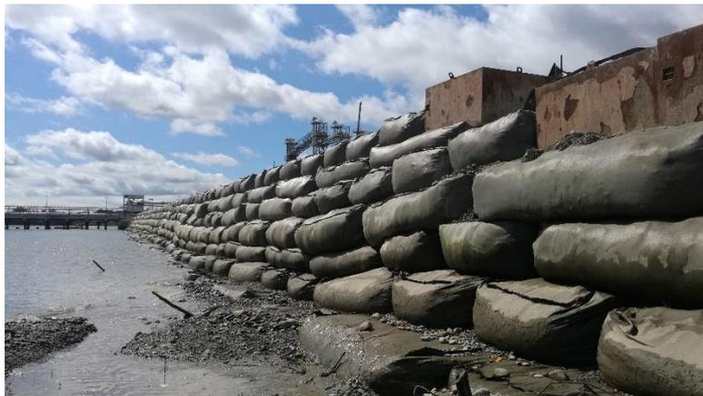
**Figure 13: Geotextile megabags retaining wall**
