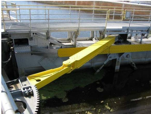
**Fig. 14: Miter Gate Strut Assembly**
