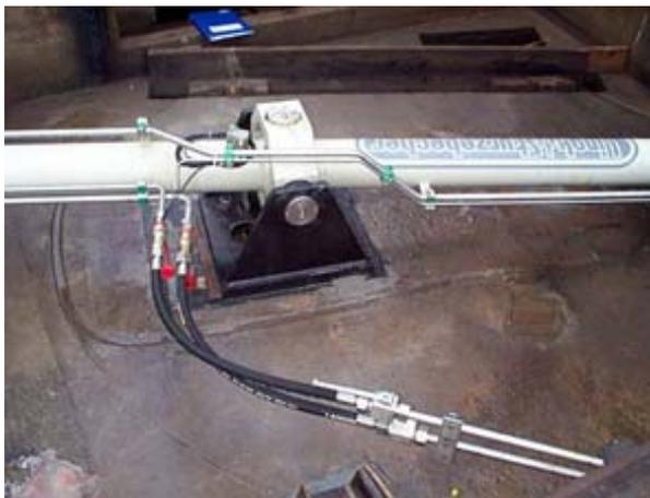
**Fig. 16: Supporting of gate cylinder for quick replacement**
