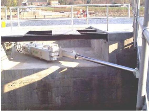
**Fig. 12: Self-Contained Drive System – United States Army Corps of Engineers Pittsburgh District**
