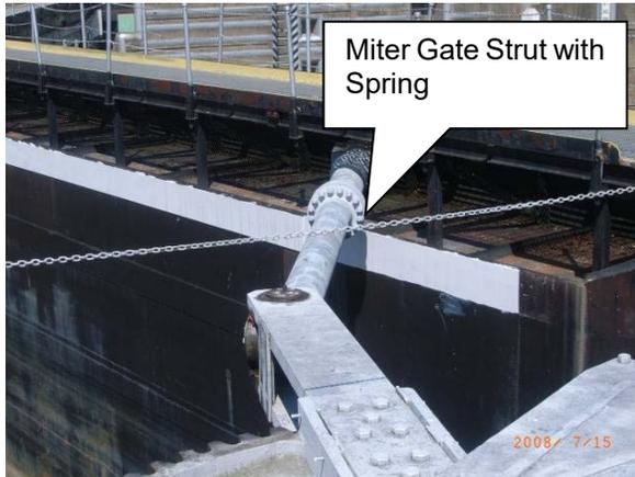
**Fig. 13: Miter Gate Strut Spring**
