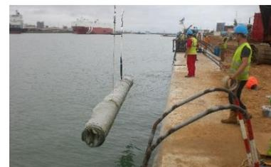
Figure 14. Lowering mattress to be rolled out by divers
