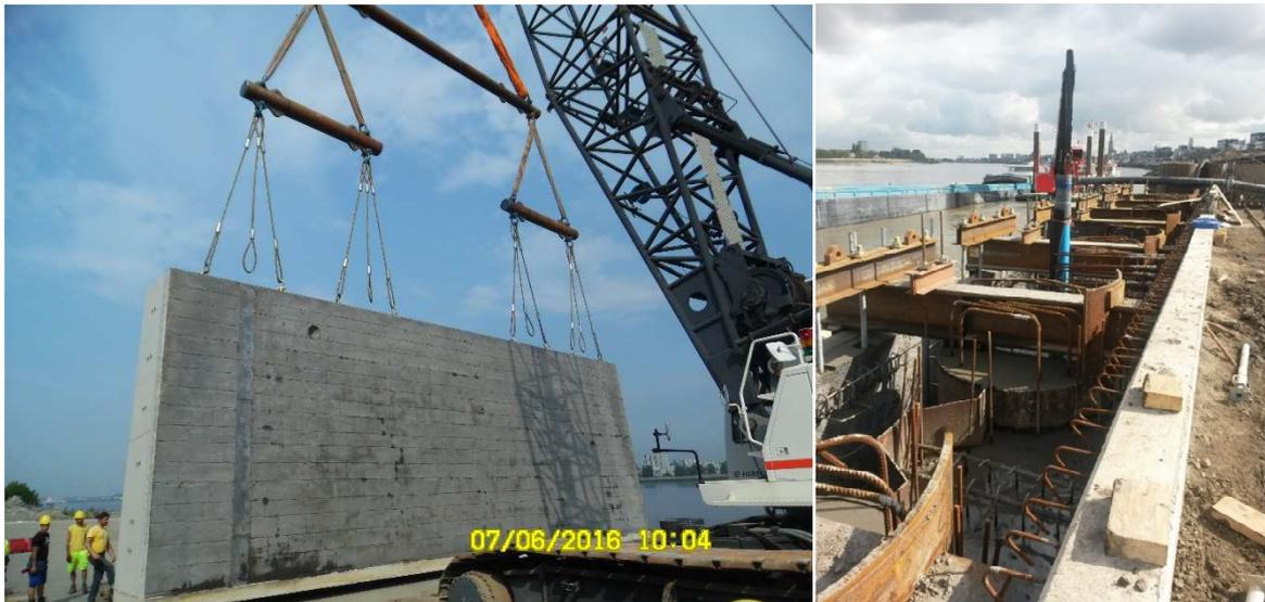
**Figure 11: Prefabricated concrete facing elements of the front wall with interconnection holes, ready for placement (left) and elements mounted on the combined wall (right)**
