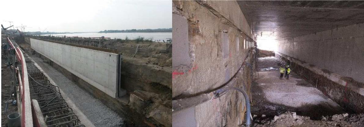
**Figure 16: View of the chamber front wall placed on the existing quay wall (left) and view inside the stress relieving chamber (right)**
