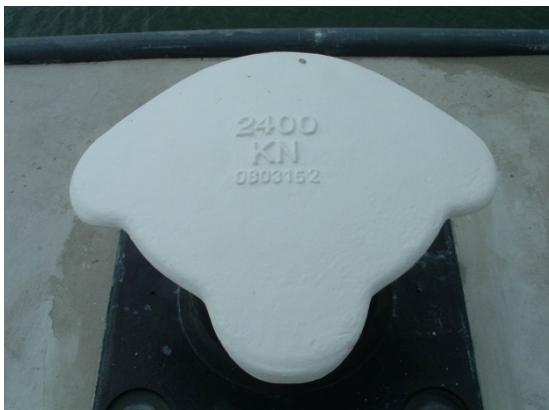
**Figure 6. Standard 2400 kN bollard Rotterdam**
