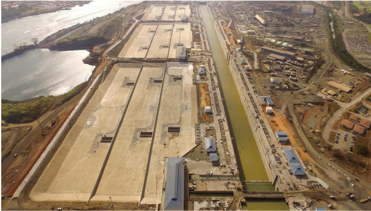
Figure 12: Pacific Complex Water Saving Basins Showing Dividing Walls and Inlets, ACP (2)
