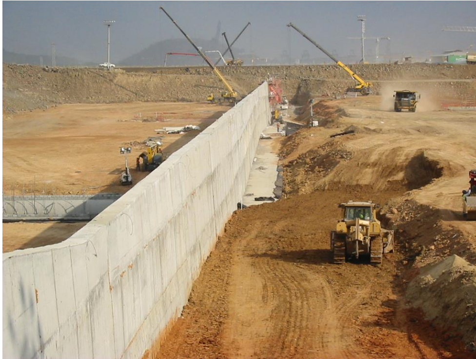
Figure 16: Dividing Wall construction, March 2015, Tetra Tech (1)
