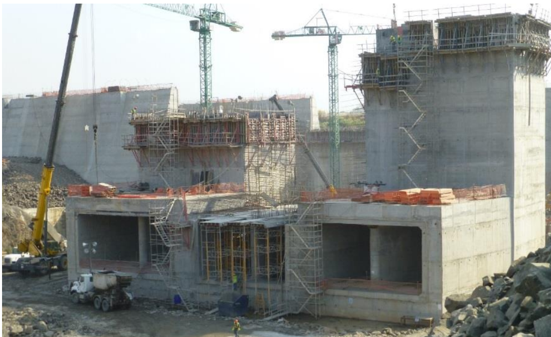
Figure 14: Valve structure under construction water saving basin side, April 2014, Tetra Tech (4)
