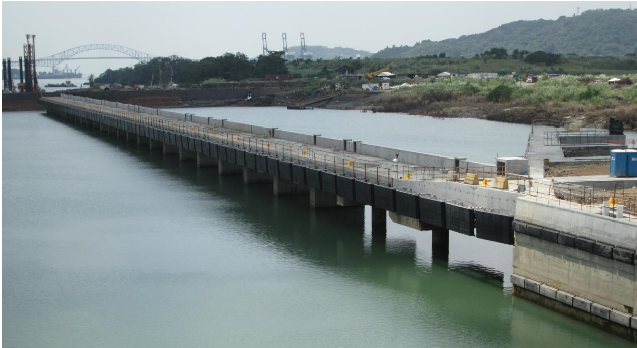
Figure 5: Pacific Outlet (Ocean) Approach Structure, Tetra Tech (1)
