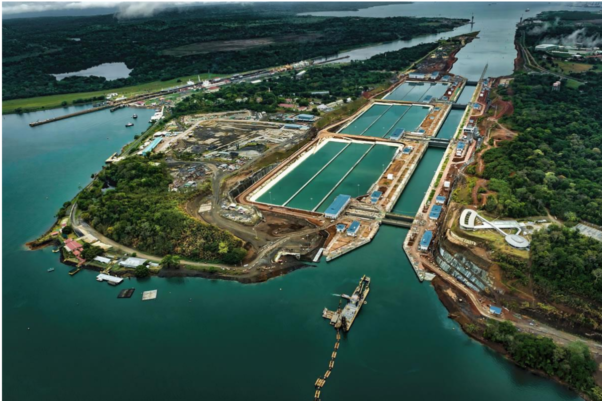
Panama Canal, Third Set of Locks, Atlantic Site, June 2016, ACP (2)
