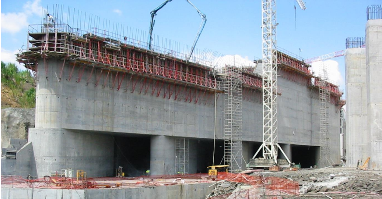
Figure 1: Pacific Outlet Monolith (Wing Wall) Construction, Tetra Tech (1)
