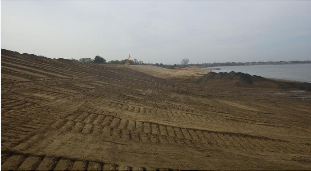
**Figure 6 - Construction of beach-fill berm**
