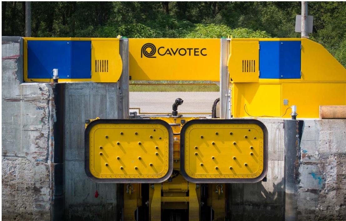
**Cavotec MoorMaster™ MM400L<sup>22</sup> system installed in the St Lawrence Seaway, Canada**
