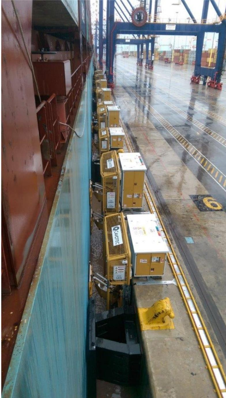
**Cavotec MoorMaster™ MM200C17 system installed in the Port of Ngqura**
