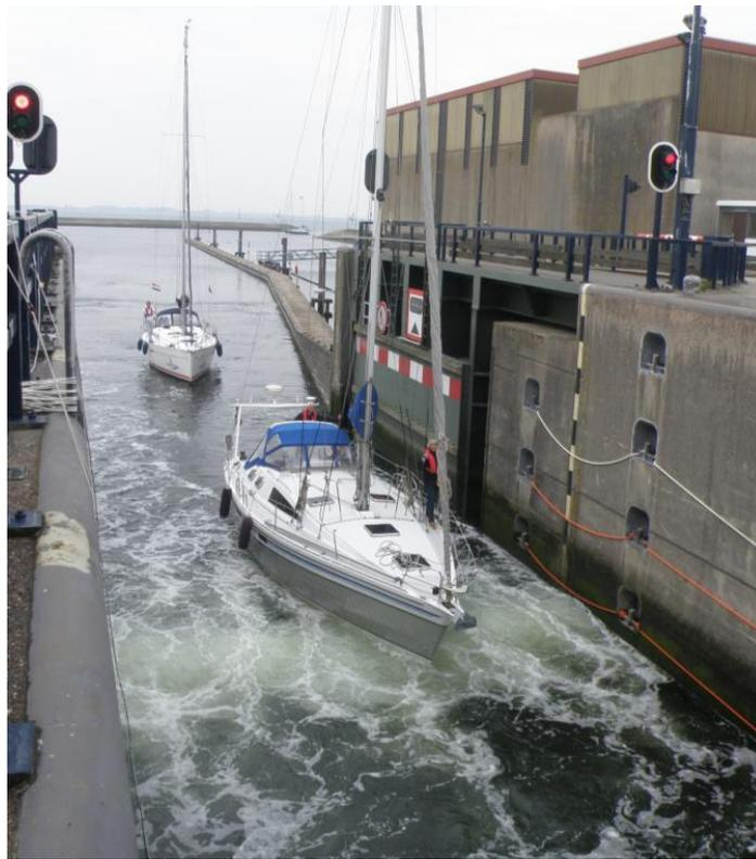
**Figure 5: Bubble screen in the Krammer recreational lock (from Weiler et al., 2015)**
